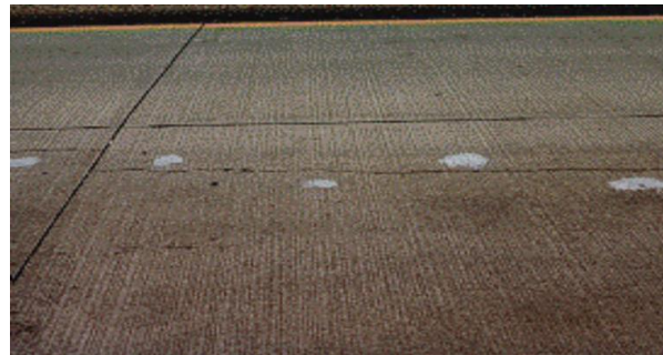
Cross Stitching Along Longitudinal Joint
