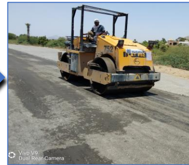
Tandem roller for sealing top layer
