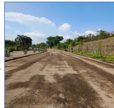
Final surface after Compaction
