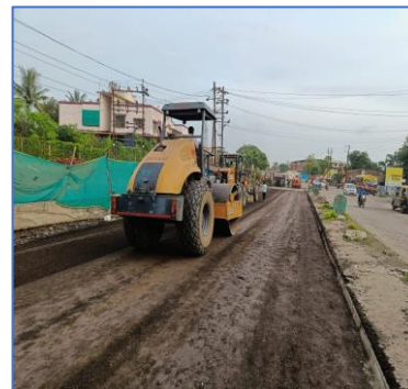
Compaction by Soil Compactor
