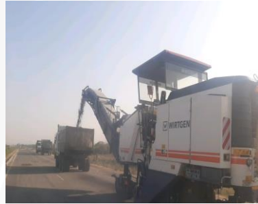
Milling Machine to mill the distressed layer
