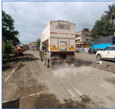
Cement Spreading by Microprocessor Controlled Spreader Truck
