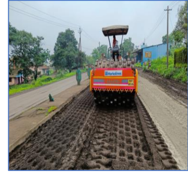
Compaction by Pad Foot Roller
