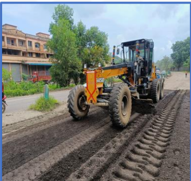
Grading & Profiling with motor Grader
