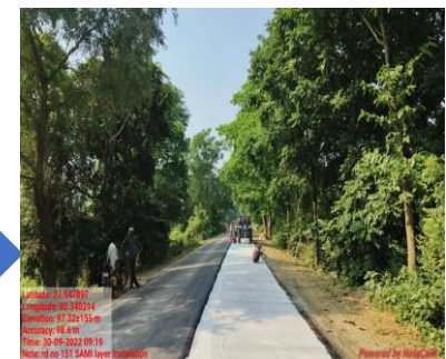
Laying of Paving fabric and Providing BC / PQC over the stabilized Layer
