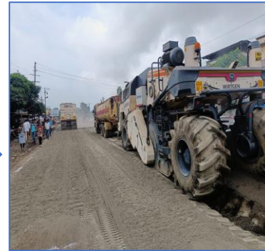
Pulverization of soil with Recycler
