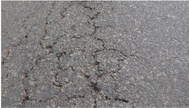
Alligator Cracks
