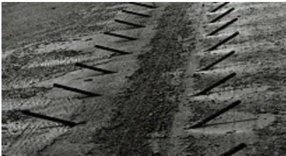
Inserting Bars along longitudinal joint
