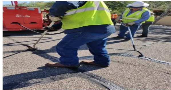
Application of hot sealant
