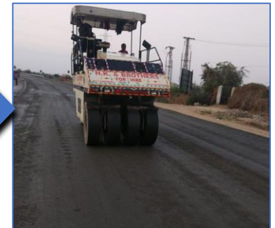
Pneumatic Tyre Roller for finishing surface
