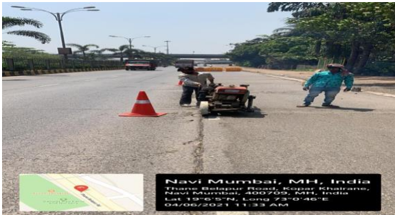
Chiselling of cracks
