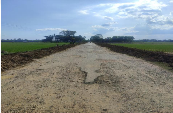
Highly Distressed/Base or Subbase Failure
