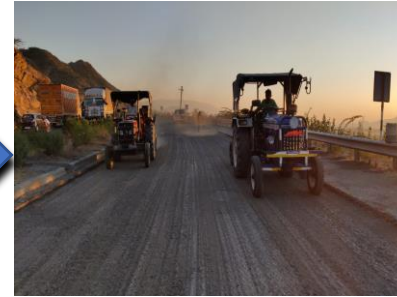
Broomer & Compressor used for cleaning
