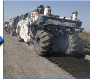
Milling & pulverisation by WR240 Wirtgen Recycler
